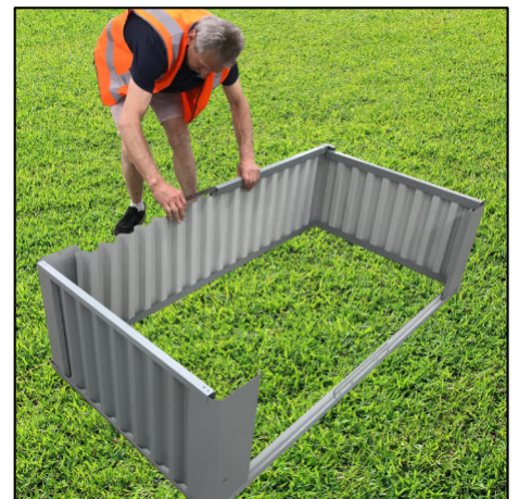
Figure 3. Securing the top rail to the wall panels, with the joiner insert in place.
